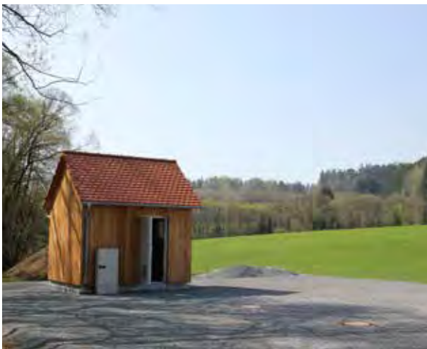
Machine house next to the plant
